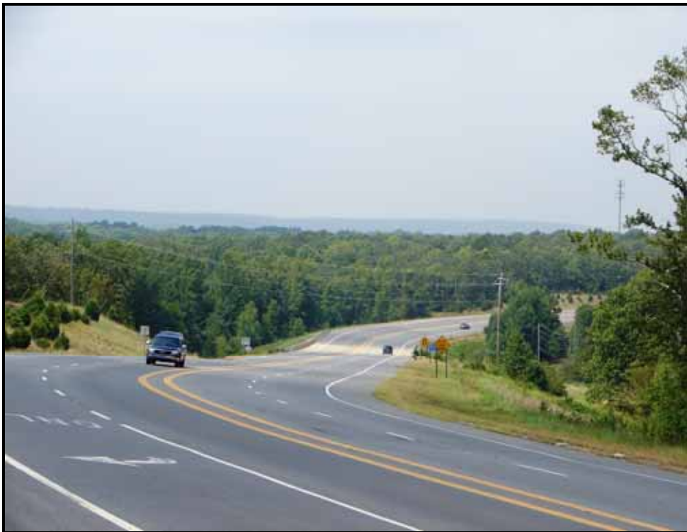
Figure 3.3-8. View south on Highway 107 from Alignment Alternative C of oak-hickory forest and the bridge over Bayou Meto.
