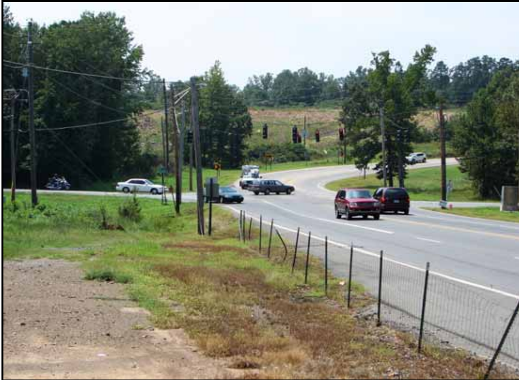
Figure 3.3-5 Intersection of Brockington Road and Highway 107.
